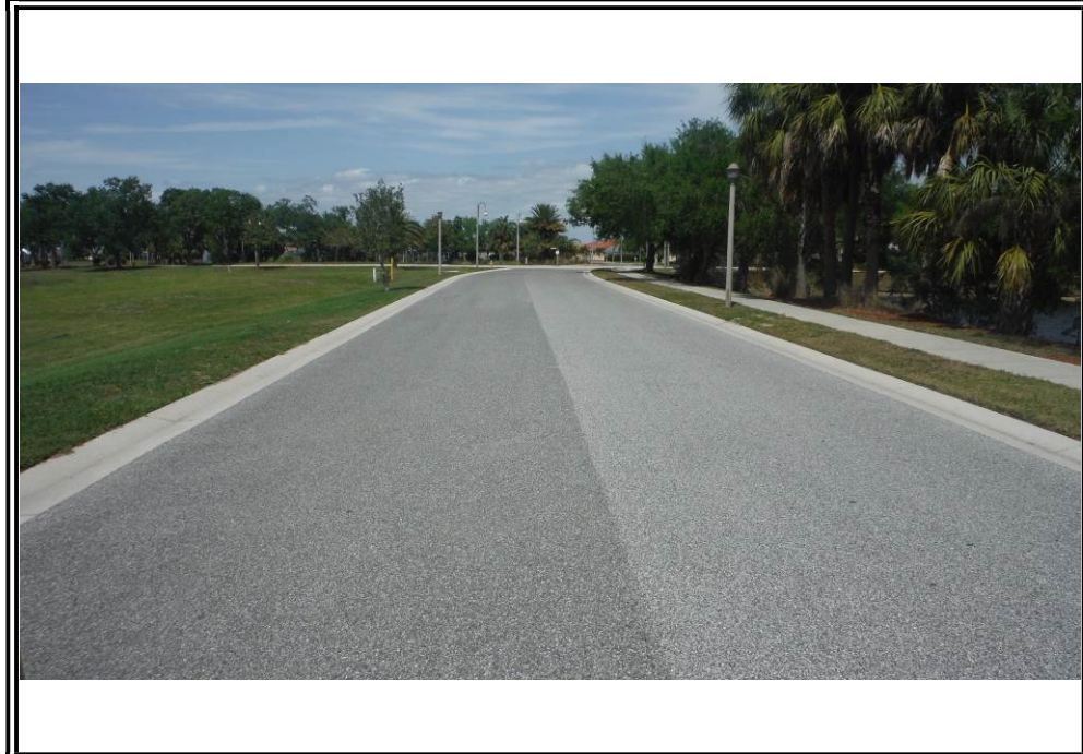
Photo No. 1 Typical Roadway Pavement Section
